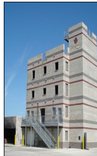
Training Tower Located at Station 1
